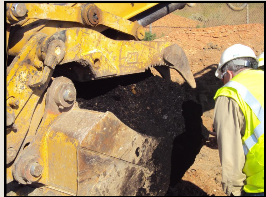
Topsoil Excavation ( ex situ )
