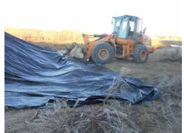
Covered stockpile of contaminated material.
