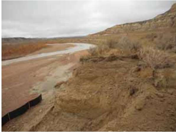
Bench excavation of the NE sidewall.
