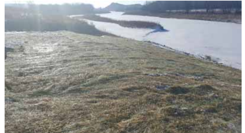
Placement of straw matting after backfilling and seeding were completed.
