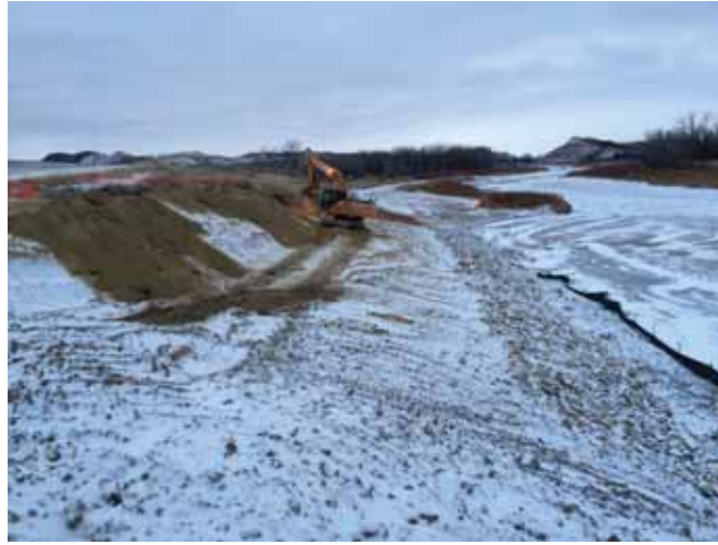
Backfilling with clay material with rip-rap placement along excavated area.
