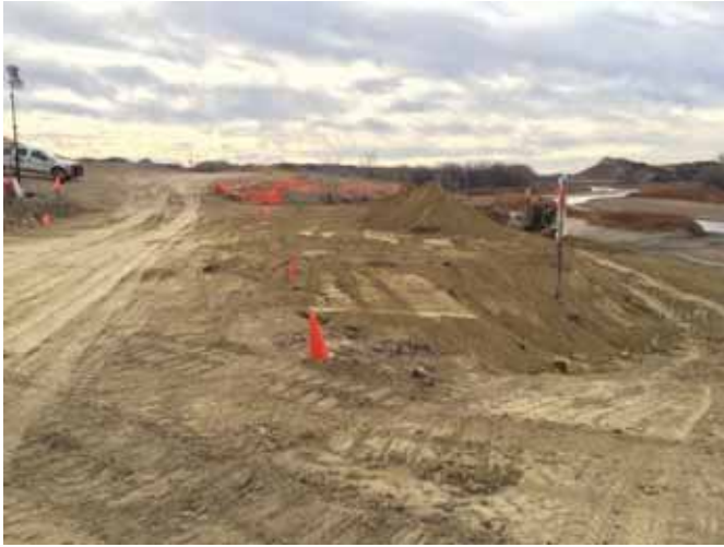
Backfilling with clay material with rip-rap placement along excavated area.
