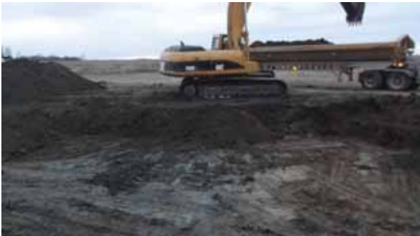
Impacted material being removed and loaded on side-dump for disposal.
