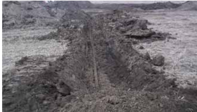
Exposed two-inch piping.
