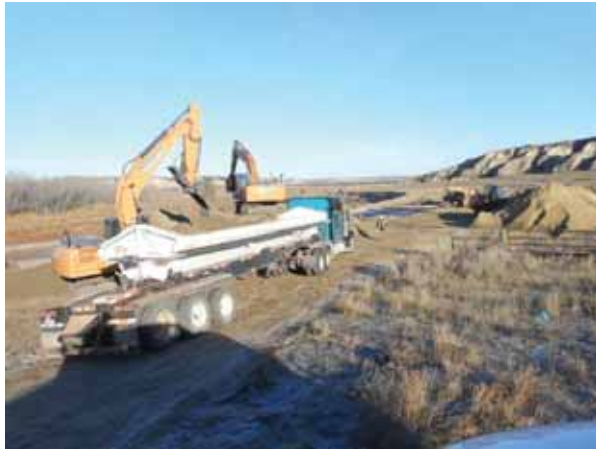
Contaminated soil being loaded for disposal.
