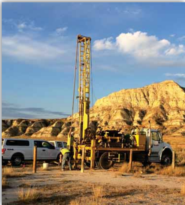
Drilling soil boring to collect soil samples and install temporary groundwater monitoring well.
