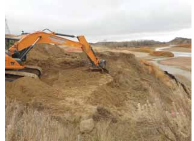
Excavation of contaminated material.
