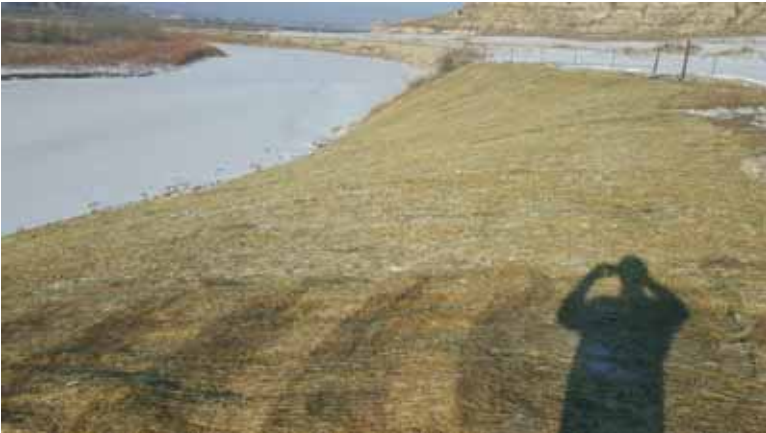
Placement of straw matting after backfilling and seeding were completed.
