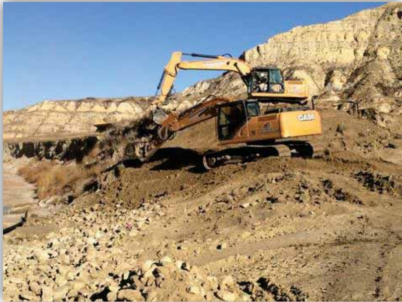
Placing rip-rap along excavated area.
