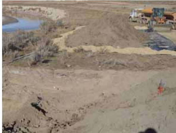
Contaminated material being stockpiled on polyethylene sheeting.
