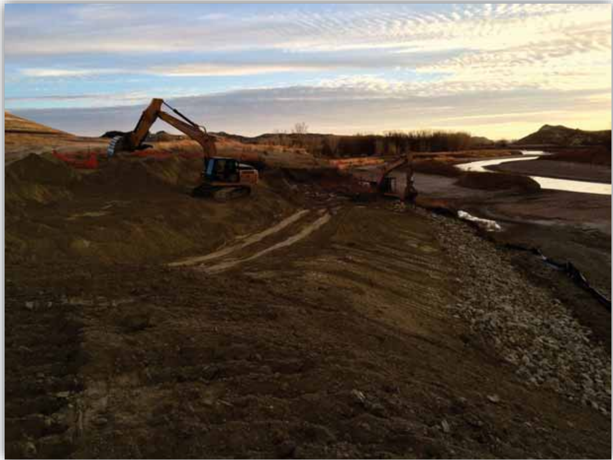
Backfilling with clay material and placing rip-rap along excavated area.
