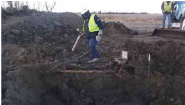
Locating extent of two-inch piping using electrical current.
